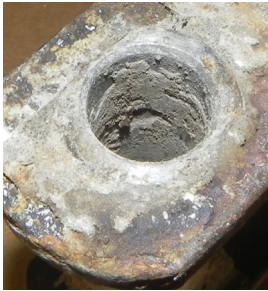
Figure 12. Heavy build-up of application material within the internal joint areas.
