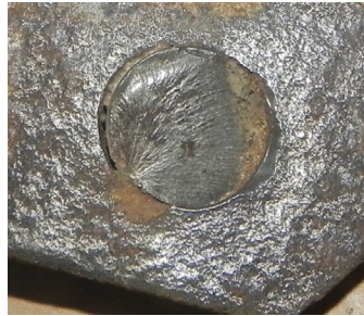
Figure 13. Corrosion pitting on the surface of the sidebar and evidence of torsional fatigue observed on the pin fracture surface on the head side.
